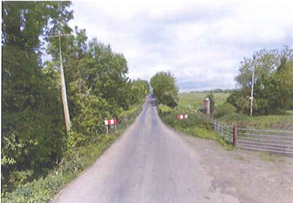
View overlooking bridge from south
