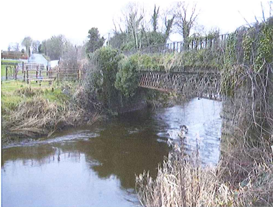
Upstream elevation of bridge
