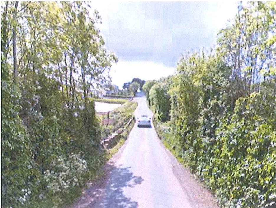
View overlooking bridge from north
